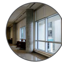
Mylar formed Concrete Columns have a stone appearance and are to be coloured to match the buff Tyndall stone of the convent
