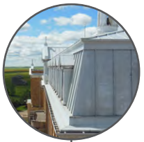
Mansard Roof white metal cladding inspired by adjacent convent materials
